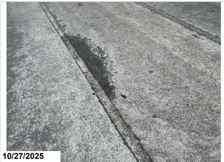
Span 1 unit 4 spall along keyway
