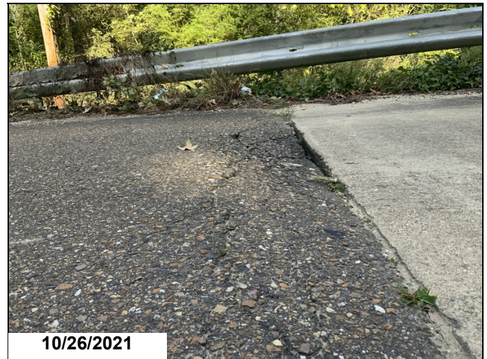
Bent 1, left lane roadway has settled.
