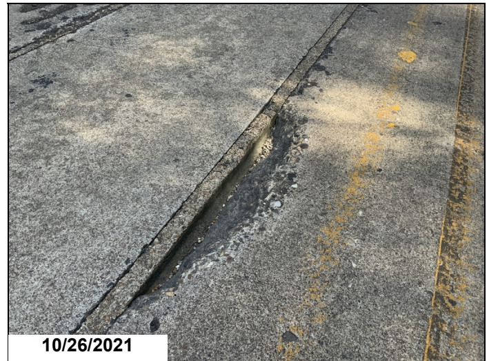
Span 1 Unit 4, at the edge of the grout keyway has a 3'x 6" spall.
