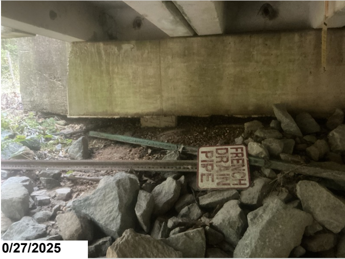
Embankment has settled for up to 8" below the cap, 6' from the right end.
