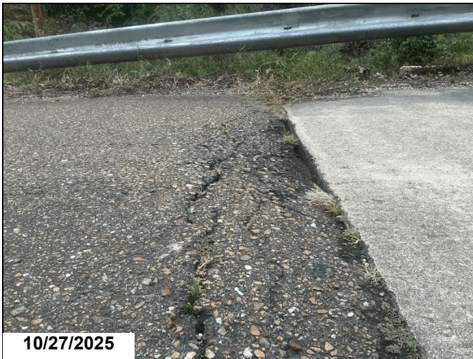
Approach at bent 1 left lane has roadway settlement
