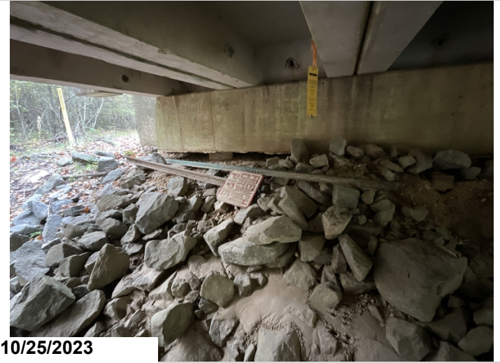
Bent 1 has settled upto 8" for 6' from right end
