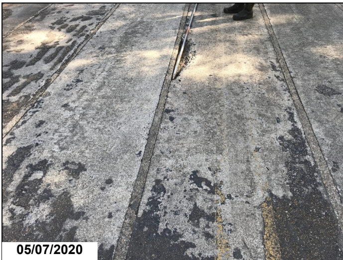
Span 1 Unit 4, 3' spall adjacent to shear key on Lt. side of the PC Unit.
