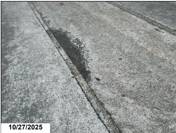
Span 1 unit 4 spall along keyway
